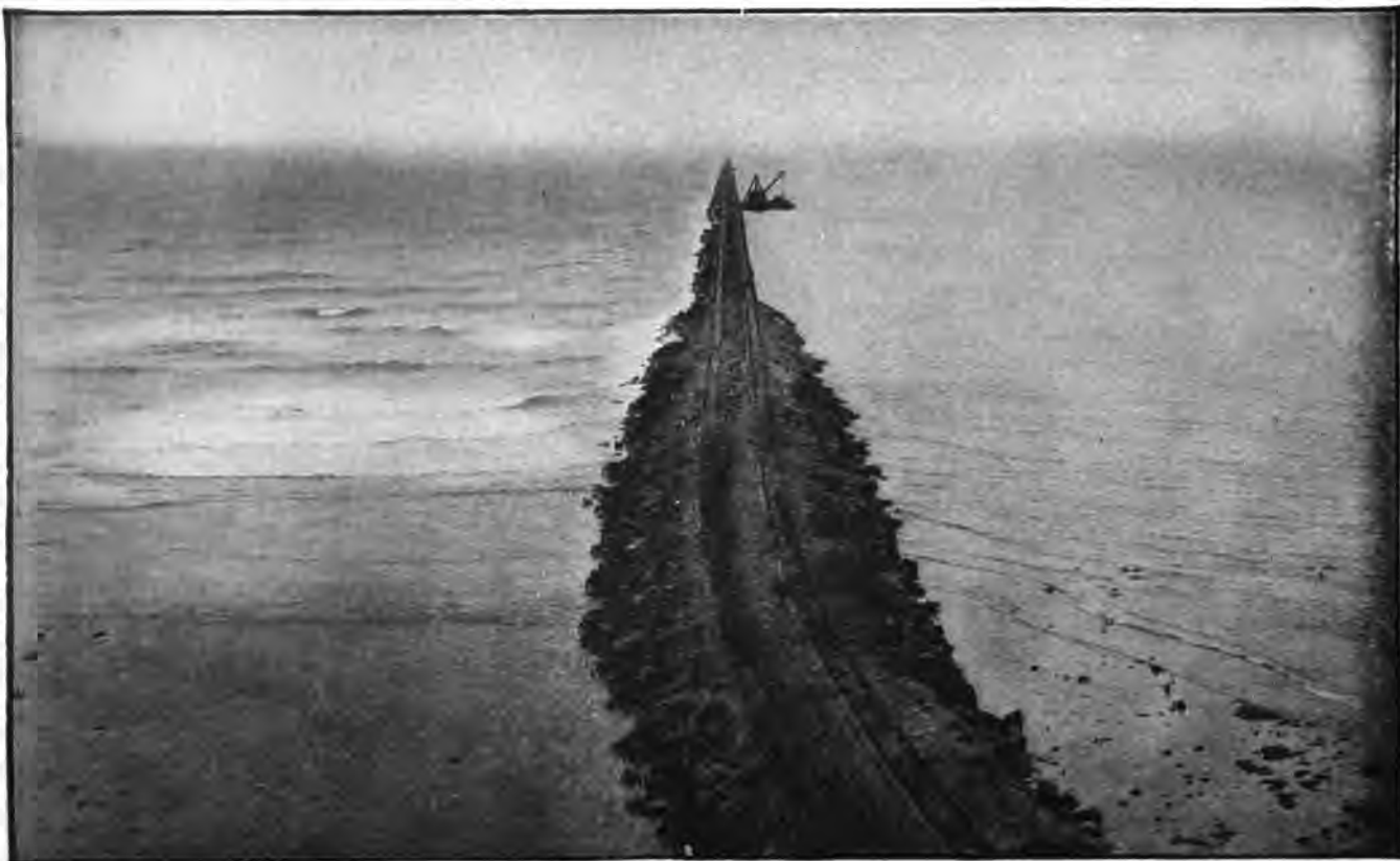
THE WEST BREAKWATER, LOOKING SEAWARD FROM TORO POINT.
